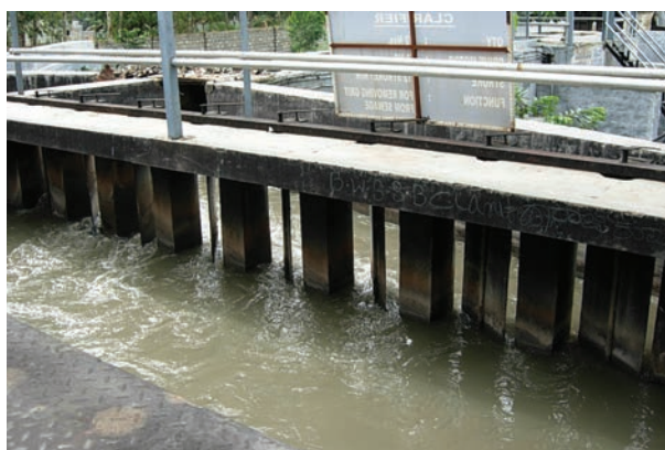
Fig. 18.4 Grit and sand removal tank
