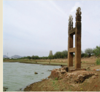
Sluice in Tank Srivilliputtur
