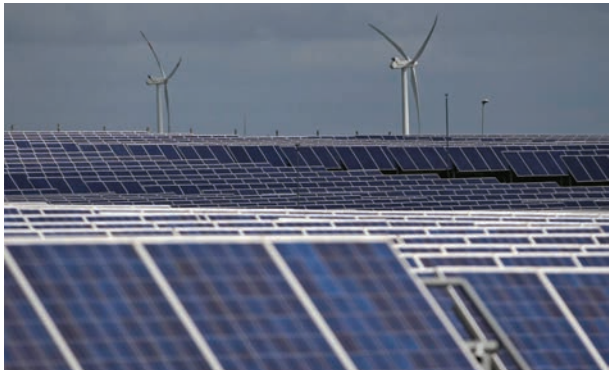
Kamuthi solar power plant
