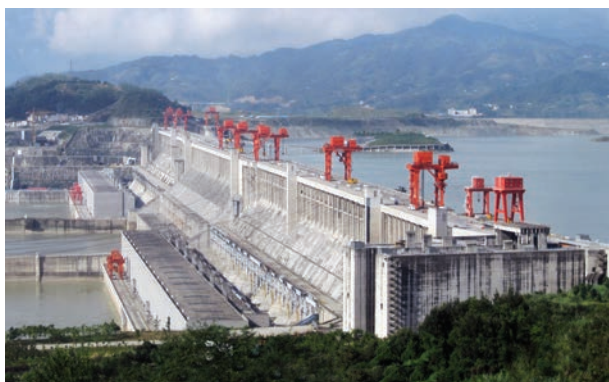
Three Gorges Dam, China
